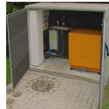
Compressed Air Flushing
