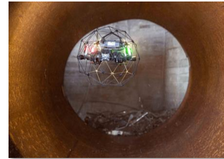
Sewer System Inspection
