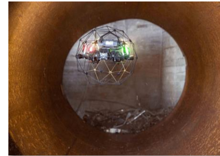
Sewer System Inspection
