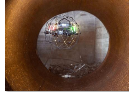
Sewer System Inspection
